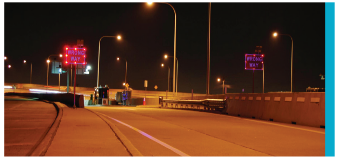
Figure 9. A Sample of Flashing LED WRONG WAY Signs at South End of Dallas North Tollway (Image: TxDOT)
