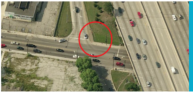
Figure 31. Right Angle Between the Left Edge of Exit Ramp and Right Edge of Crossroad (Image: Bing)
