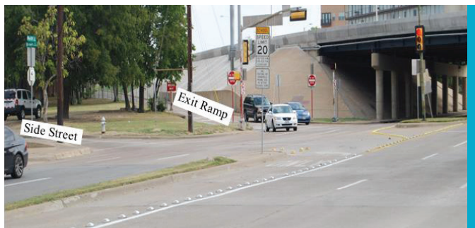
Figure 13. NTTA Southbound Exit Ramp at Wycliff Avenue, Before Median Enhancement (Image: Yang Ouyang)
