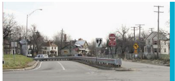
Figure 30. Median Barrier (Guardrail) Blocking View of Entrance Ramp Throat (Morena and Leix 2012)
