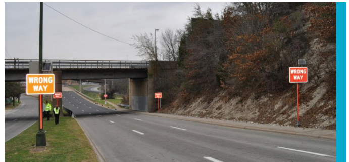
Figure 23. Three Pairs of Large WW Signs by NTTA (Image: Huaguo Zhou)
