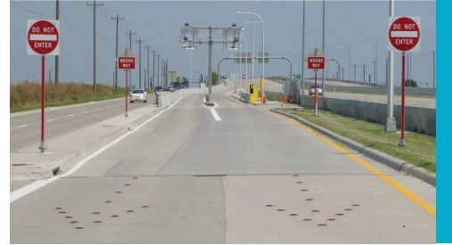
Figure 11. NTTA Exit Ramp with Red Retroreflective Strips on Sign Supports and Red RRPM-supplemented Wrong Way Arrow Pavement Markings (Daytime)
