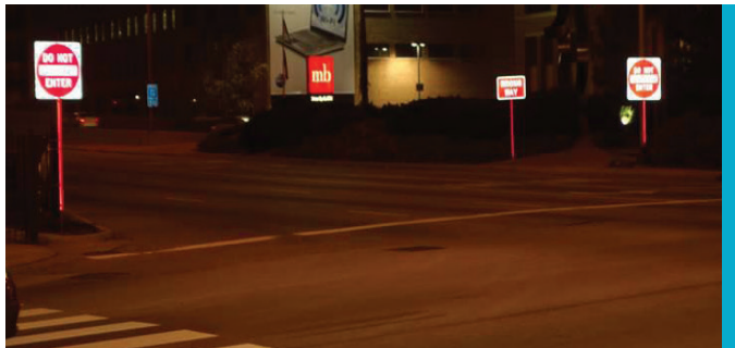
Figure 10. Red Retroreflective Tape on the Sign Post to Enhance Nighttime Visibility (Image: Huaguo Zhou)
