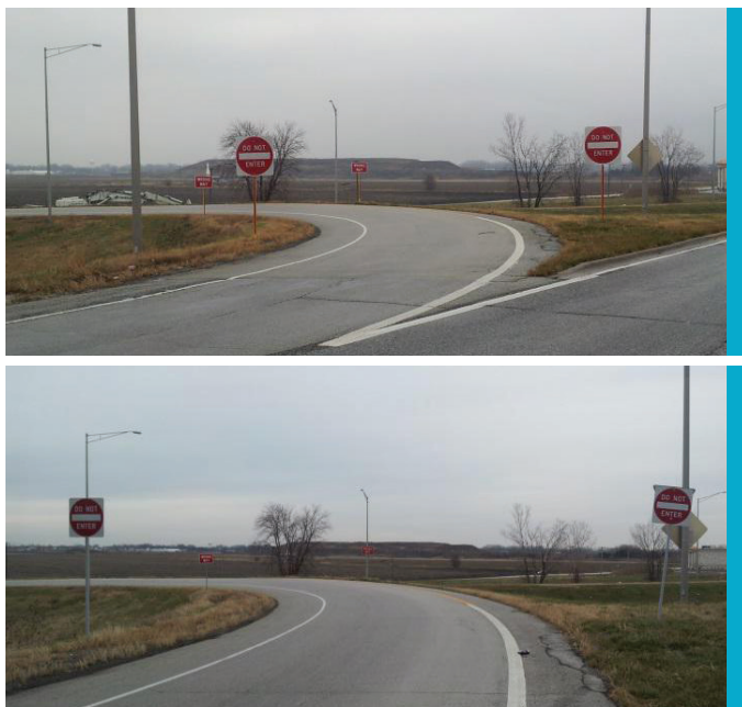
Figure 22. Before (top) and After (bottom) Pictures of DNE Signs at I.L. 394/US 30 (Image: Regina Cooper)
